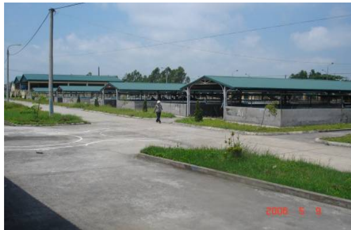
Concrete fish growing tanks
