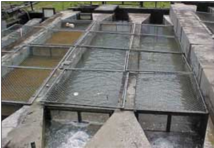
Figure 3. Parallel type of raceway tanks for trout culture at the Fisheries Research Centre at Trishuli, Nuwakot
