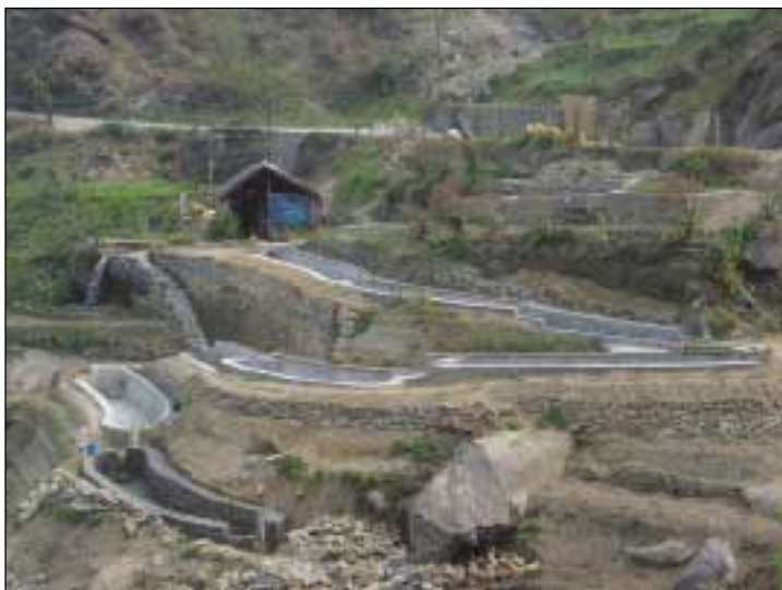
Figure 4. Linear type of raceway tanks for trout culture built by a farmer to fit the available landscape
